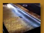
We use Astro-foil (R-15) insulation along the entire length of the floor. Plus an additional wrap around the holding tanks
